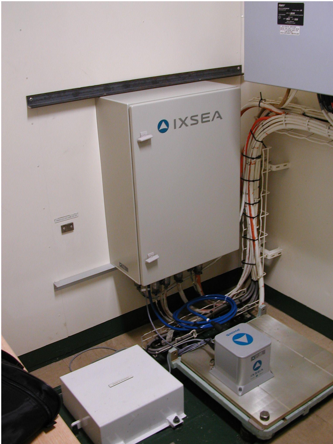
Figure 2 - Installation in replacement of old mechanical gyro (retrofit): Aluminum interface plate
